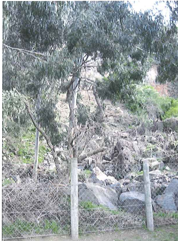
Photo 3-2 – Boulders at the Base of Catch Fence post the September Earthquake.
