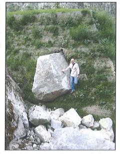
fully serviceable condition. More importantly, the embankment continued to remain in a serviceable condition after three other large falls, each of approximately 3000 tonnes. Maintenance was recently carried out on these embankments and the works comprised removal of accumulated fallen material and the cosmetic (plus very minor structural) repairs to the surficial portion of the embankment.
