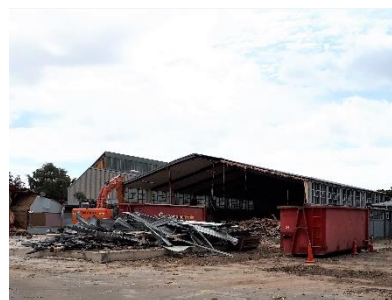
Image: Linwood College demolition
